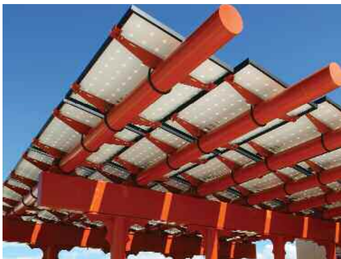
Solar panels at Zocalo's Solera, Denver
